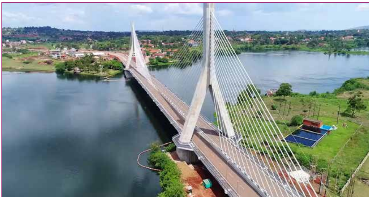
Top-down development? The newly constructed Nile bridge in Uganda
